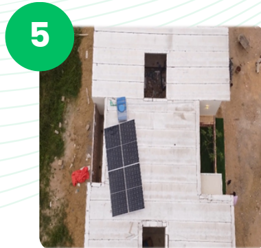
5 Solar and MEP system is installed
