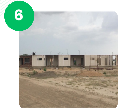
6 Completing any interior elements required
