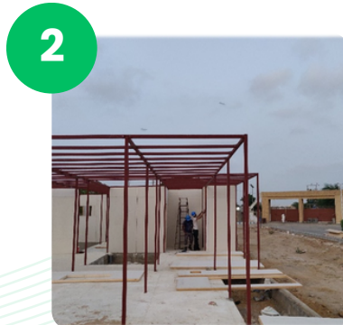
2 Steel structure is assembled
