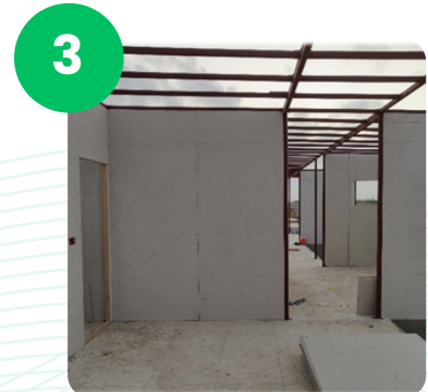
3 Wall panels are attached
