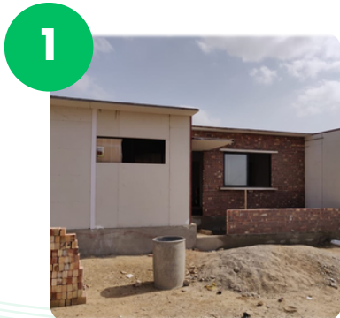
1 Installation of plumbing system and civil works
