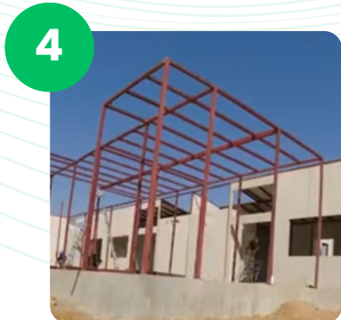
4 Placement of roofing components
